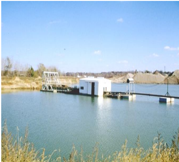
Sand and gravel pumping operation
