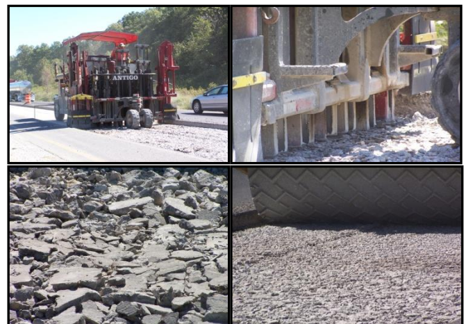
Rubblized In-place Concrete
