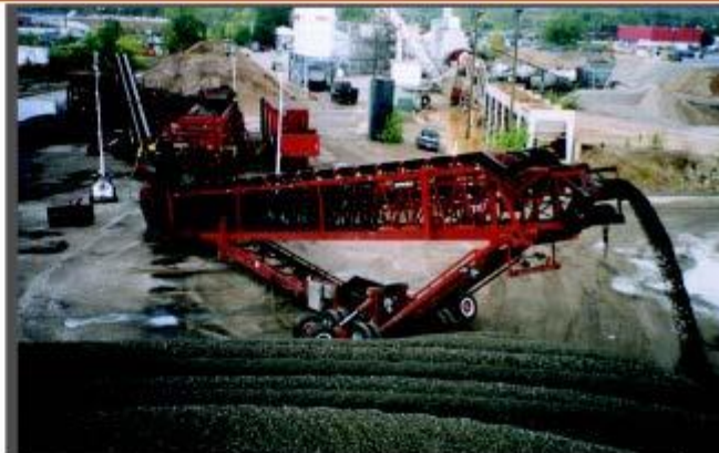
WINDROW STOCKPILING WITH A TELESCOPING CONVEYOR F21
